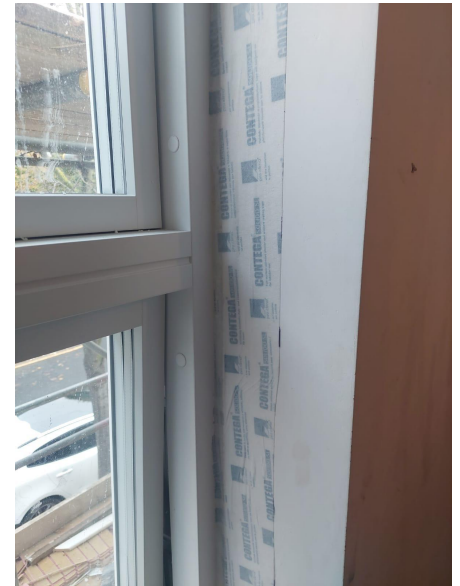
internal airtight tape for airtightness
