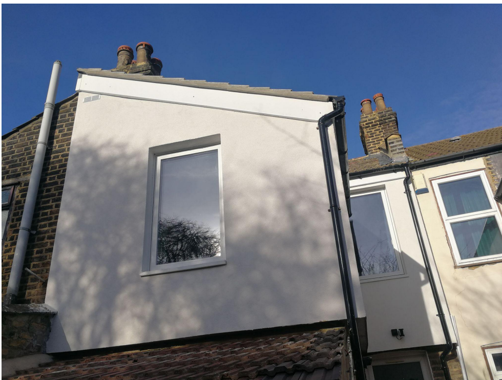
Rafters & verge extension to allow for EWI. 100mm blue XPS over rafters insulated roof. Longitudinal battens to allow for ventilation, under roofing felt. Black XPS on face and underside of verge extension
