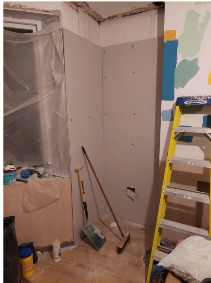
NE corner - Aerogel IWI required on party wall + front wall to mitigate thermal bridge
