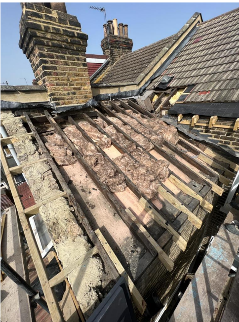
verge & eaves timber extension
