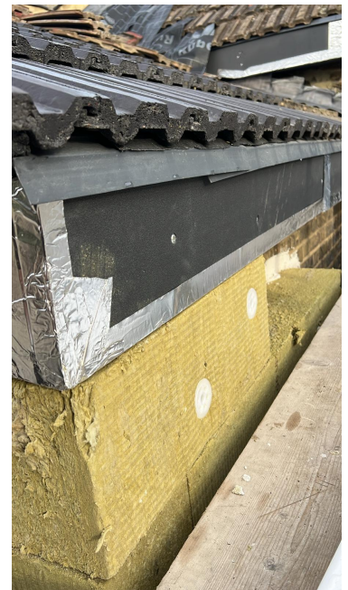
thermal continuity with eaves, verge & EWI
