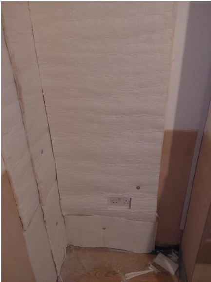
NE corner - Aerogel IWI required on party wall + front wall to mitigate thermal bridge
