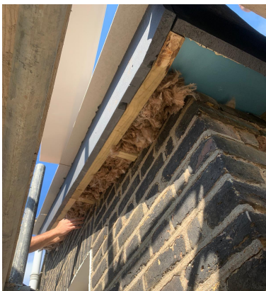
Rafters & verge extension to allow for EWI. 100mm blue XPS over rafters insulated roof. Longitudinal battens to allow for ventilation, under roofing felt. Black XPS on face and underside of verge extension
