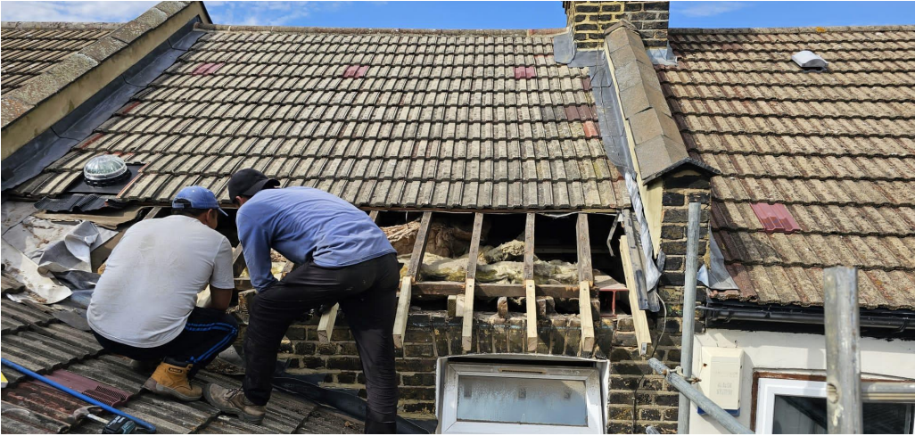
rear main roof with eaves extension
