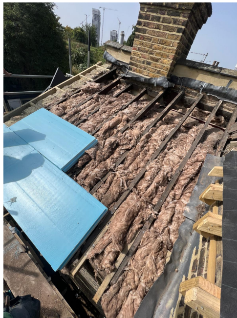
100mm blue XPS over rafters insulated roof.
