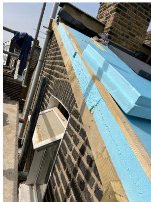
Rafters & verge extension to allow for EWI. 100mm blue XPS over rafters insulated roof. Longitudinal battens to allow for ventilation, under roofing felt. Black XPS on face and underside of verge extension
